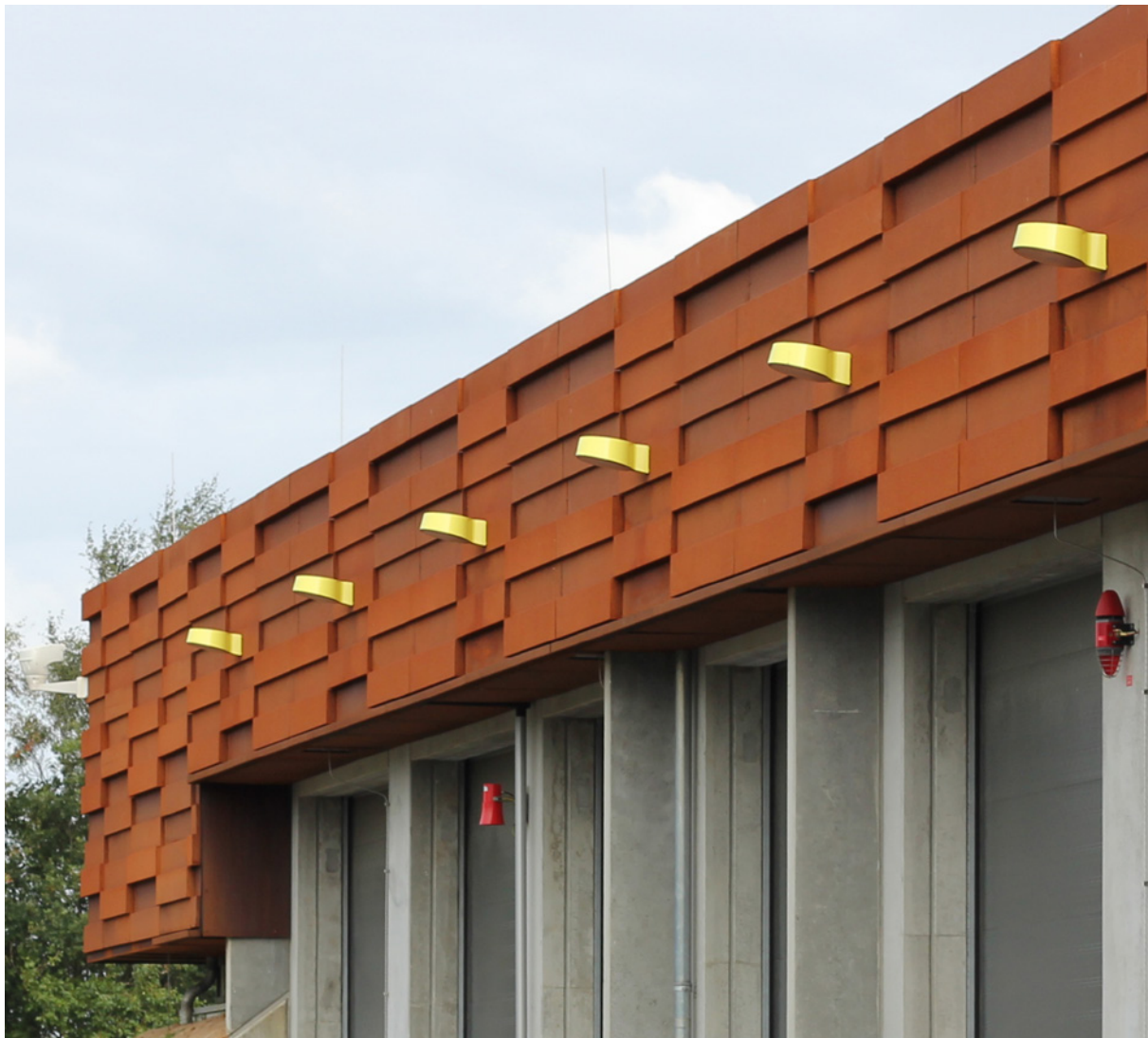
Egtved Gas Compressor Station, architects: C.F. Møller
